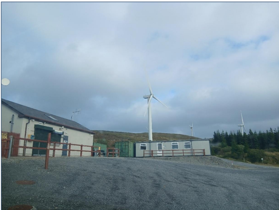
Plate 6-15 Existing Wind Farm infrastructure classified as Buildings and artificial surfaces (BL3) recorded throughout the Proposed Wind Farm.
