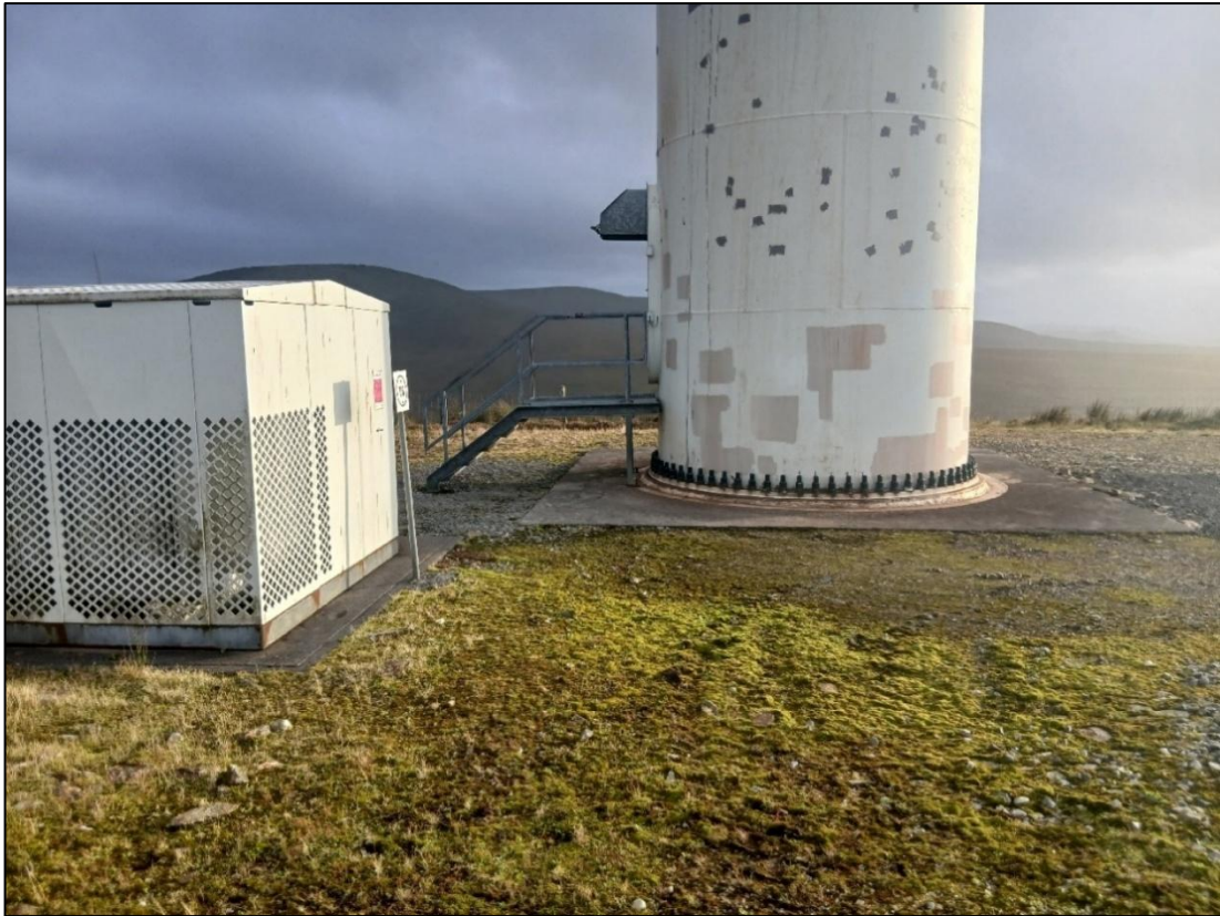
Plate 6-14 Existing Wind Farm infrastructure classified as Buildings and artificial surfaces (BL3) recorded throughout the Proposed Wind Farm
